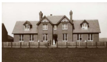
Southwold Community Hospital
