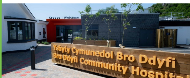
BRO DDYFI COMMUNITY HOSPITAL IN NORTH WALES
